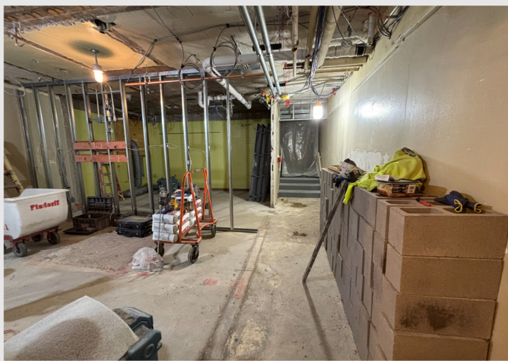
Wall framing, rough-ins, and blocking in place in the Lower-Level Flex/ELL Rooms. Masons are ready to starting laying the block walls!
