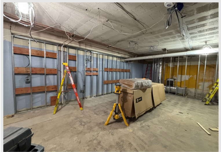
Wall structures are in place in the Lower-Level OT/PT Room as well, along with the new unit ventilator staged up for install!
