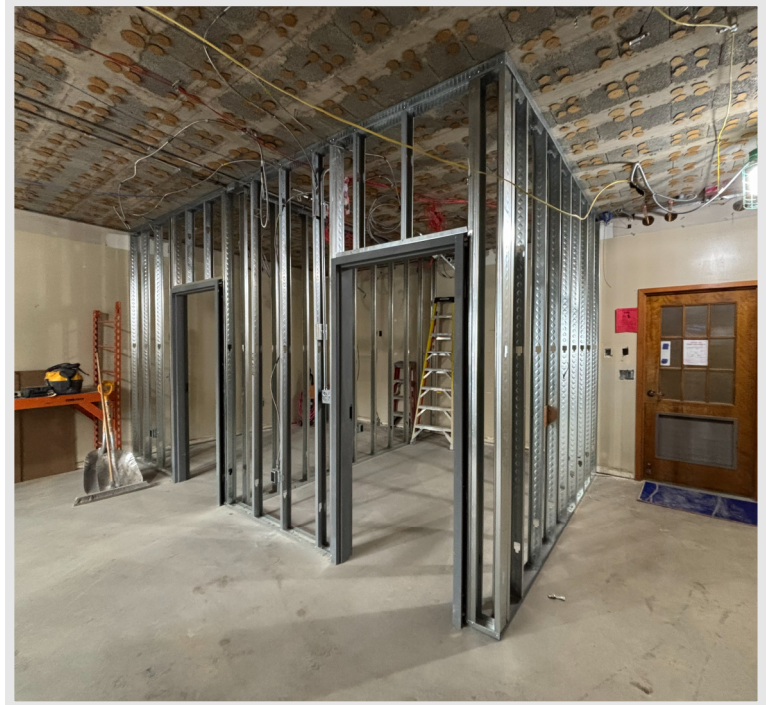
Wall framing and early rough-ins in place creating the structure for the SGI Rooms in the main Speech Office on First Floor!
